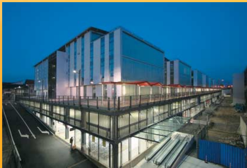
The new Turin headquarters
